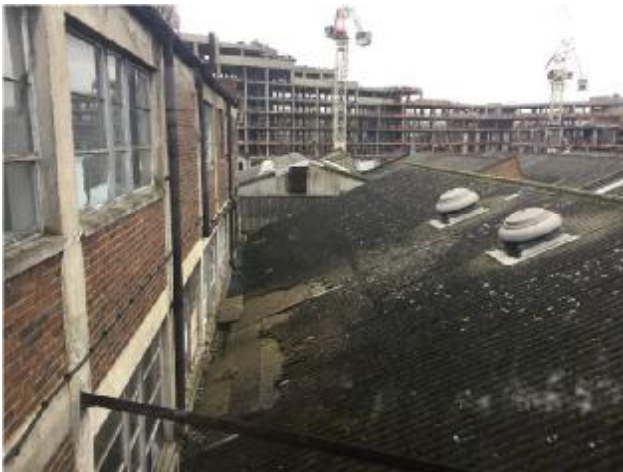
7. Building 1 (middle) - Example of damage to roof covering
