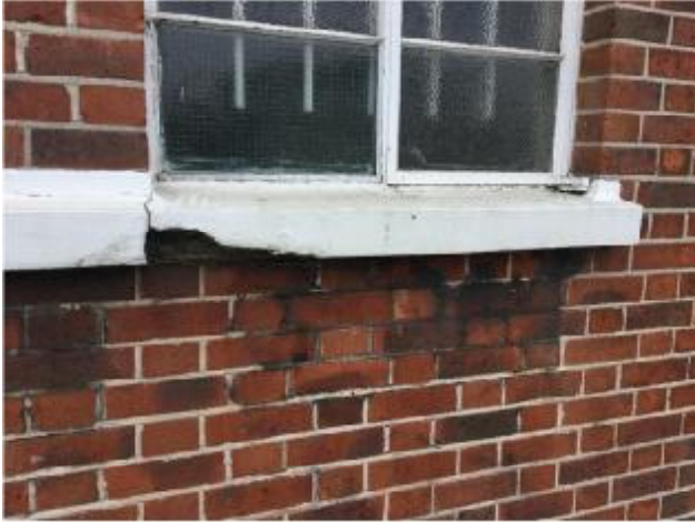
29. Building 2 (front) - Example of damaged window sill
