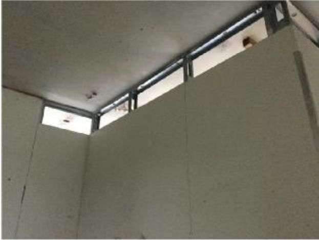
17. Building 1 (rear) - Example of incomplete studwork partition
