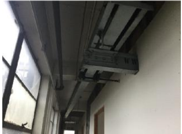
20. Building 1 (rear) - Hoist built into studwork partitions
