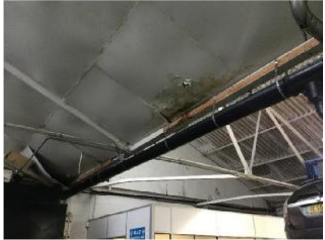
38. Building 2 (middle) - Example of roof leak
