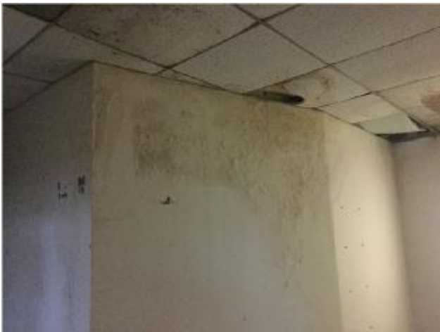
27. Building 2 (front) - Damp to office wall
