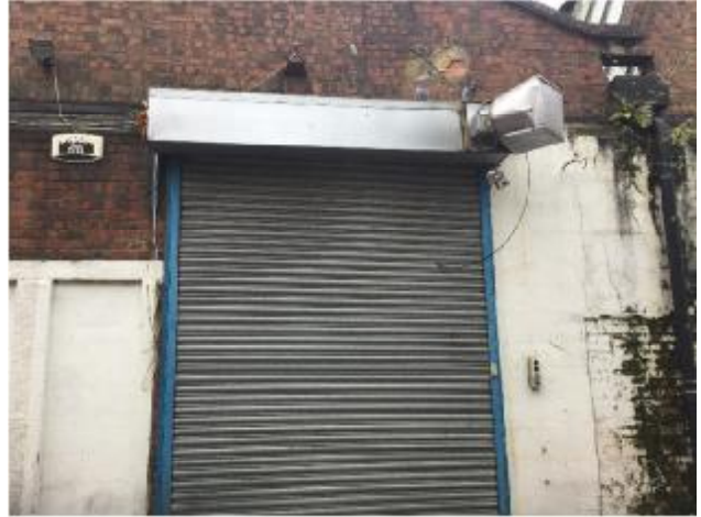
10. Building 1 (middle) - Example of roller shutter door
