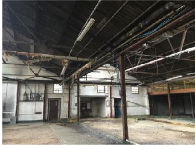
6. Building 1 (middle) - Example of corrosion to steel frame
