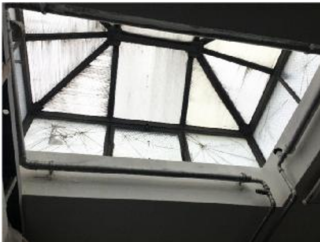
15. Building 1 (rear) - Damaged lantern light to flat roof
