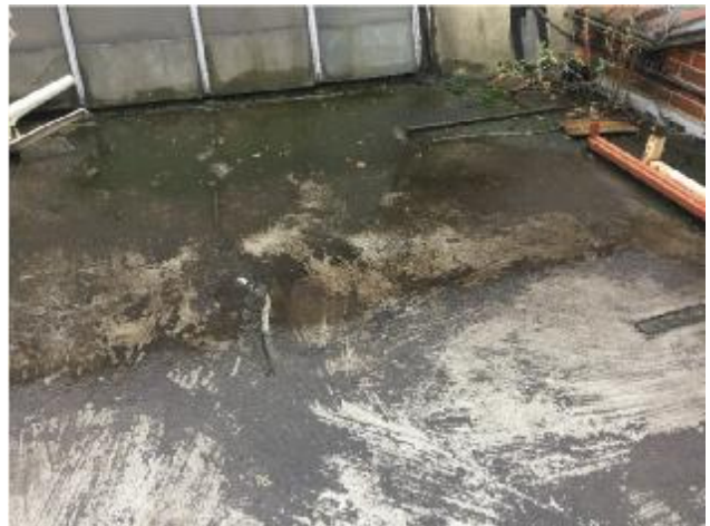
32. Building 2 (front) - Lower flat asphalt roof
