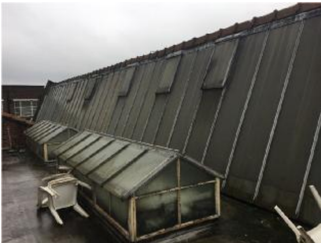
31. Building 2 (front) - Lantern lights to lower flat asphalt roof
