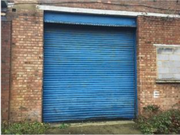
37. Building 2 (middle) - Example of roller shutter door
