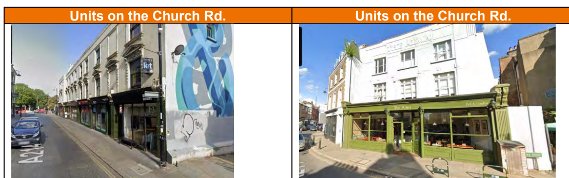
Figure 1-8 Examples of retail units Crystal Palace District Centre
