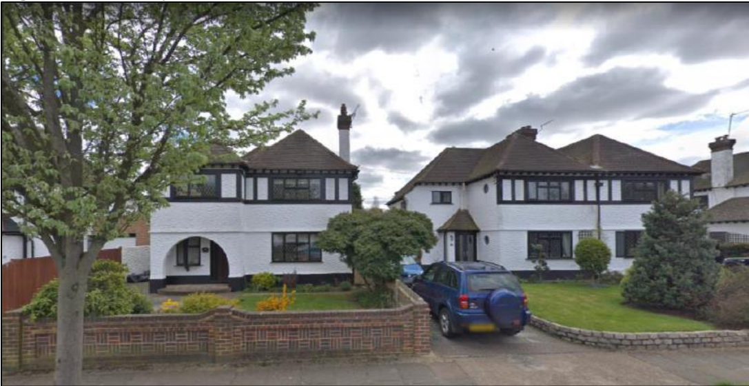
Figure 8: 5-9 Ladywood Avenue, north-west elevation
