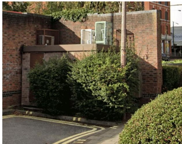
Figure 9 - Harwood Avenue automatic monitoring station
